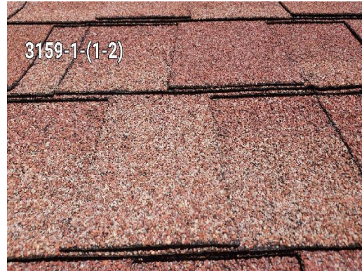
3159-1 Asphalt Shingle/Red, Tar/Black Typical Exterior Roof
