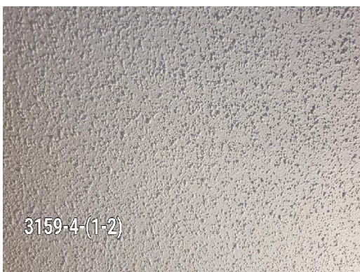
3159-4 Ceiling Surfacing Texture/Cream (2% Chrysotile) Typical Interior Ceilings
